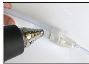
6. Use a heat gun to seal the heat shrink tube.
